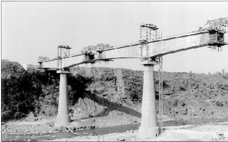
The Tawi bridge of the JURL project
