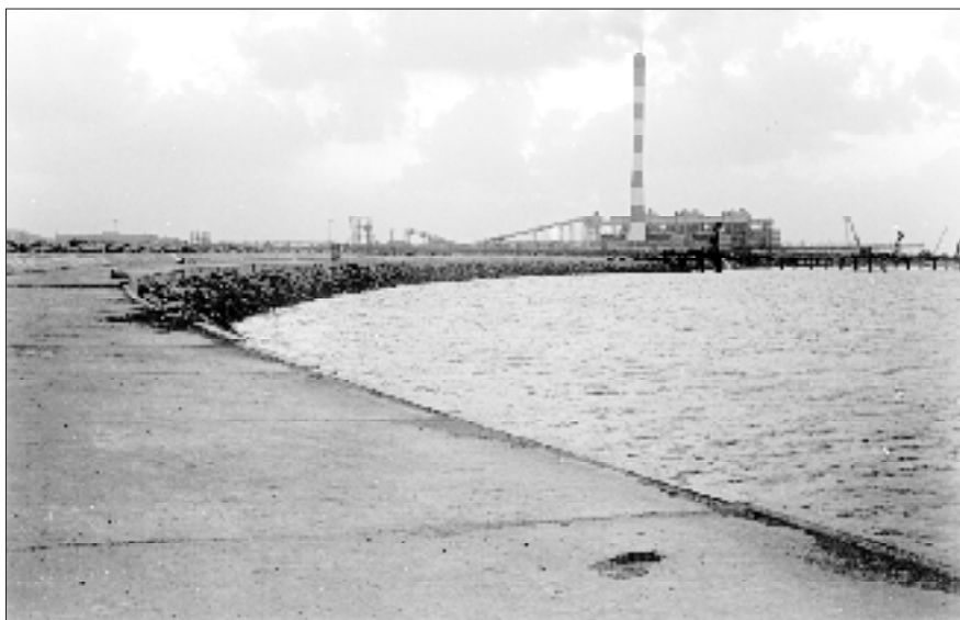
Construction of breakwater, Ennore Coal Port project, Tamil Nadu
