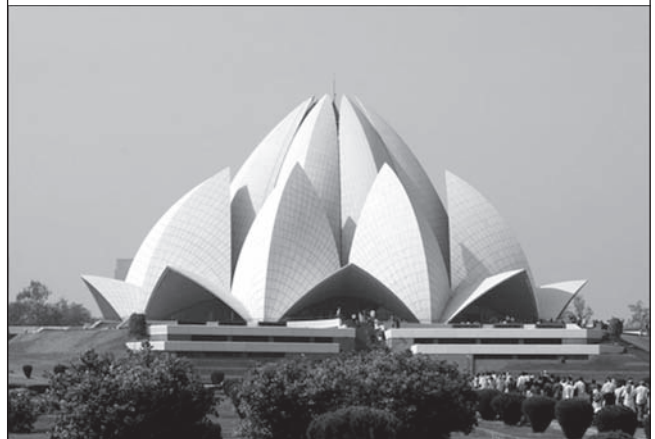
(c) The Bahai Temple in New Delhi, designed by Architect Fariborz Sahba
