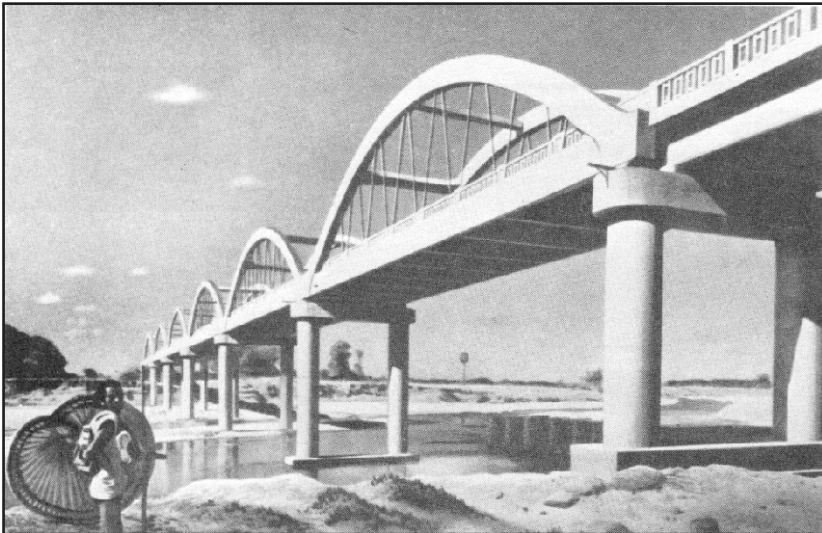
13 - The Bonum River Bridge on the Jharsuguda-Sambalpur road has six bowstring girders with inclined hangers.
