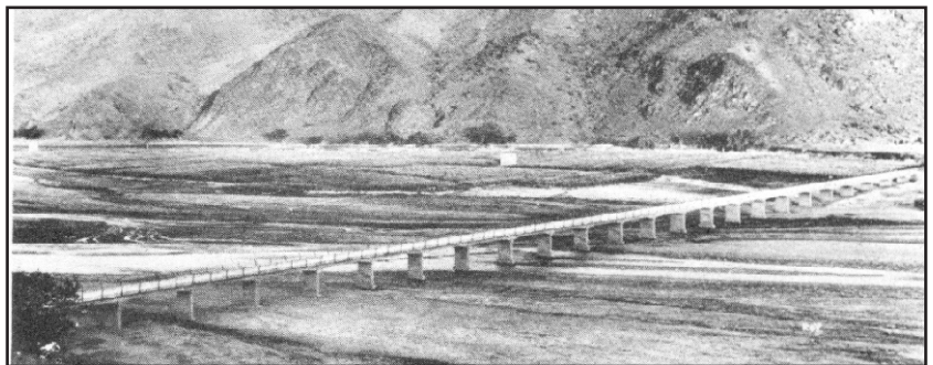
14 - The Boya Bridge, a submersible structure with continuous spans.
