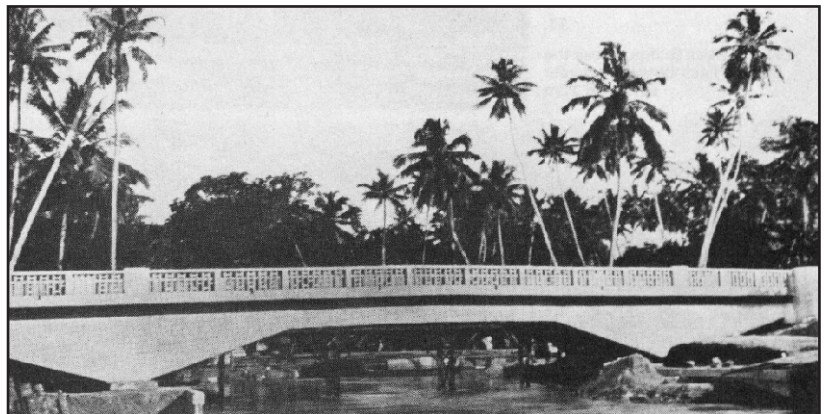
6 - The Kayenkulum Bridge has hollows in the cantilevered sections which are filled with sand.
