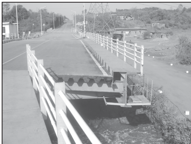
Figure 9. The other arm of the bridge being opened
