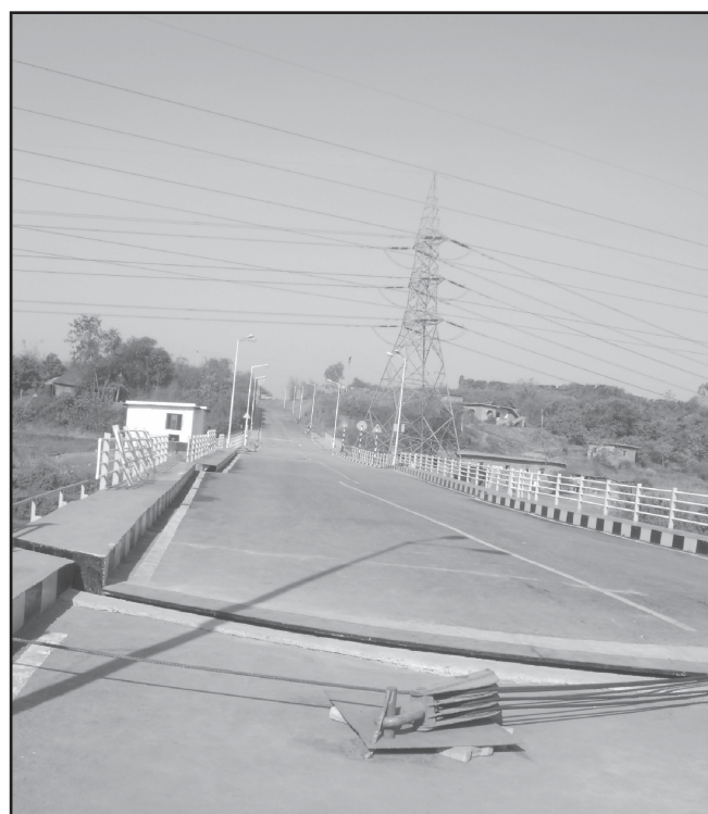
Figure 4. Completed bridge from Poira side
