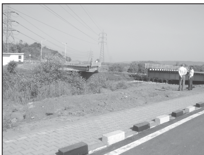
Figure 10. The other arm of the bridge fully opened
